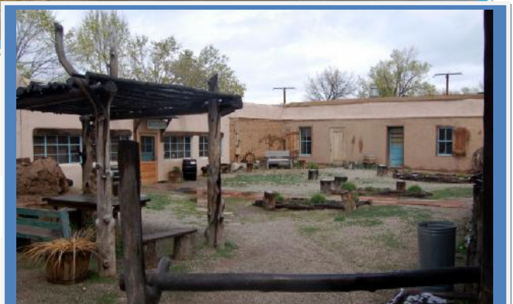
The rear courtyard
