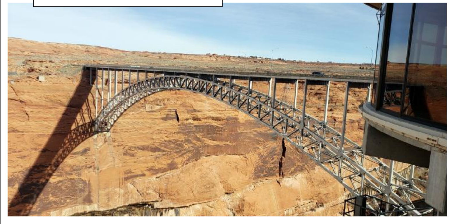
The vehicle bridge across the gorge
