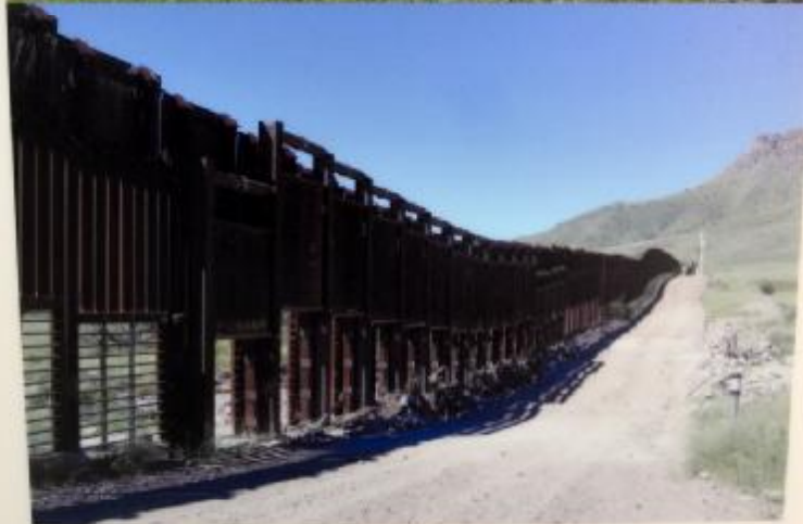
There are places along the fence that open seasonally to allow floodwaters to flow through. There are other special openings where wildlife can cross.
