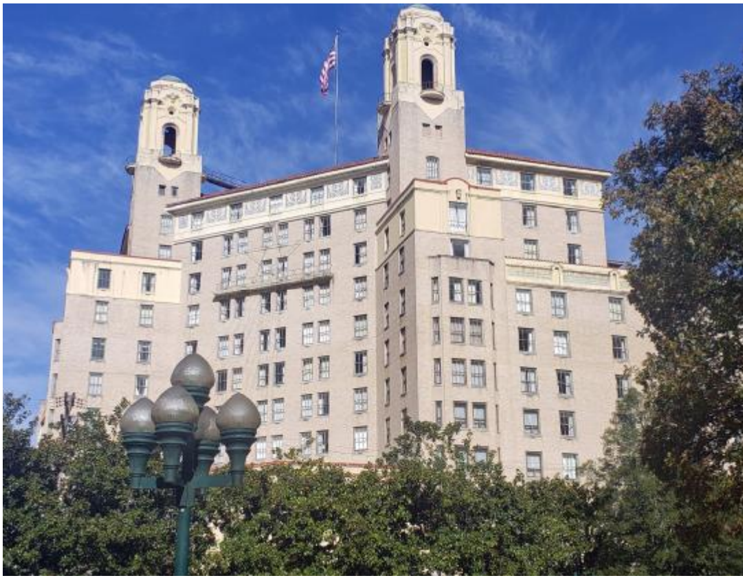
The Arlington Hotel – Probably the most famous hotel in Hot Springs and the most rebuilt – This is the third version (fire).
