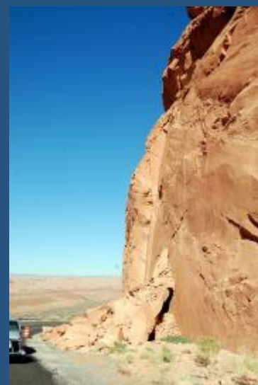
Looks like a recent landslide
