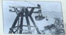
View of towers and cables from the Ermita Valley.
