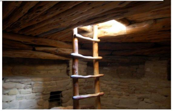
This is the only Kiva that white men are allowed access to, the reason being that it has been desanctified and is no longer used for Hopi ceremonies. It was warmer inside. Note the opening to the rear. This is actually the air inlet. The fire was built in the middle of the floor and the vent provided cold air into the Kiva and forced the smoke out the chimney hole in the roof, exactly where the ladder is. This is also the only entrance to the Kiva.
