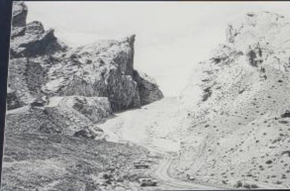
Excavation begins through the Reef. Courtesy: Emery County Sheriff's Department.
