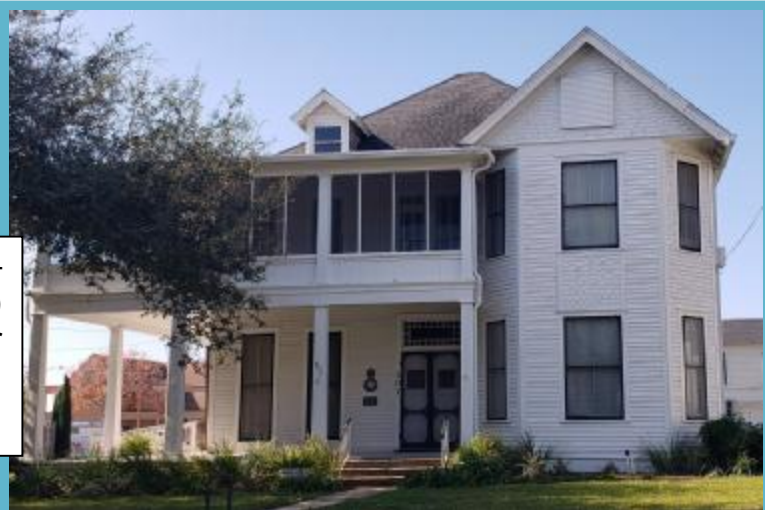
Edward Power House 1894 – His daughter Helen (one of five) married Robert Hughes Welder from the house above in 1912. Divorced in 1921.
