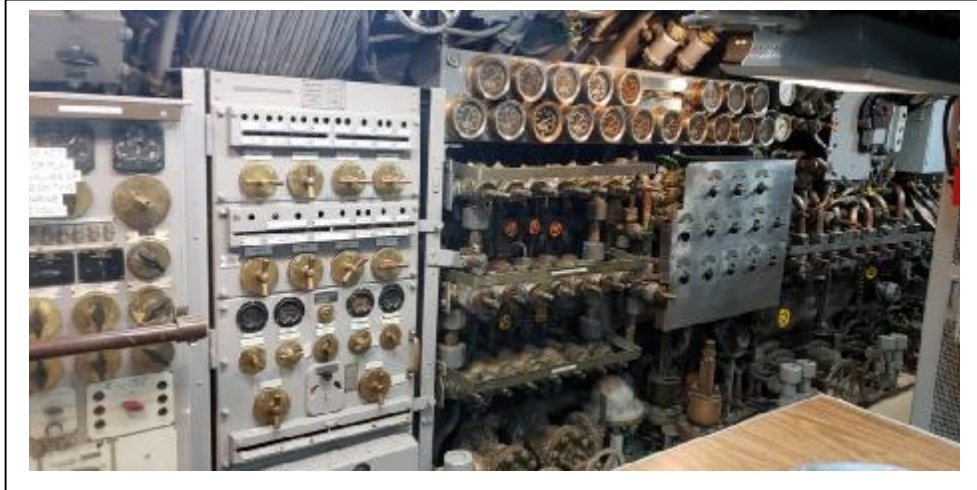
The control room, above and below
